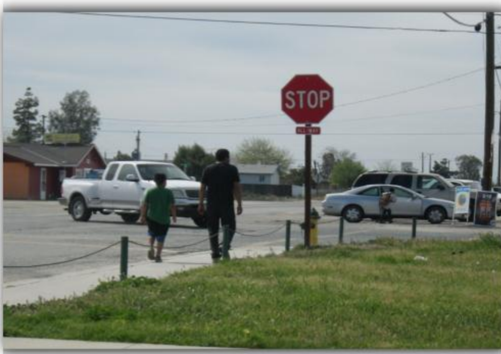
Figure 6: Sidewalk improvement proposed at Avenue 54 at Tule Road, Existing sidewalk is less than 3 feet wide and not in compliance with ADA standards. Westbound view.
