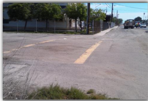
Figure 5: Sidewalk improvement proposed at Avenue 54 at Lake Road, Existing sidewalk is less than 3 feet wide and not in compliance with ADA standards.
