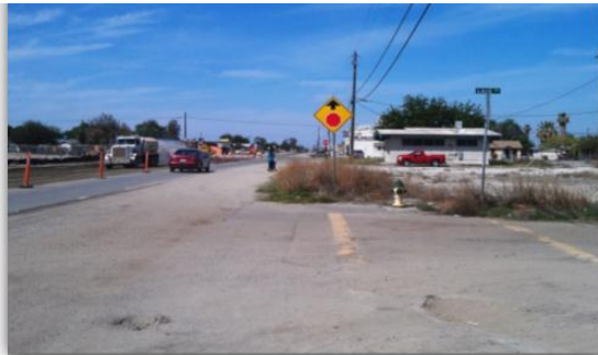
Figure 4: Sidewalk improvements proposed at Avenue 54 at Lake Road. No sidewalk to differentiate from road, making current state a potential hazard for pedestrian and children walking to school.
