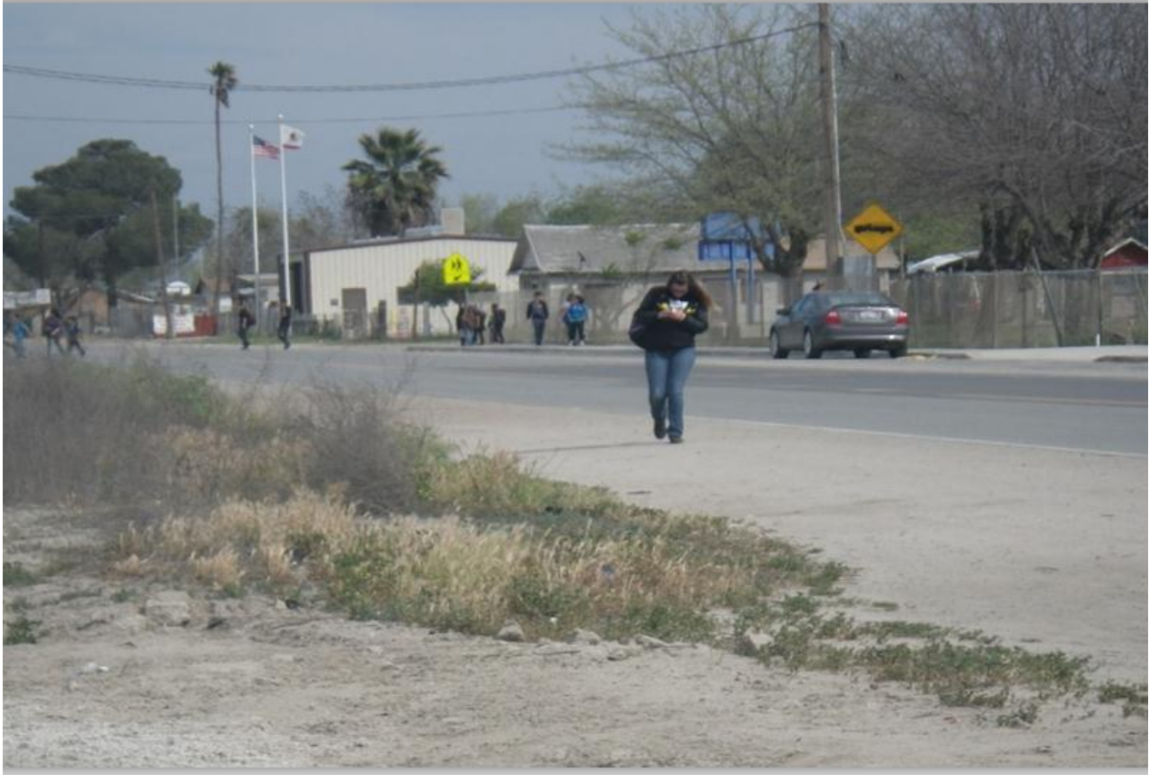
Figure 3: Avenue 54, between Lake Rd and Wilber. Sidewalk is non-existing to differentiate from roadway. Sidewalk, curb, gutter, asphalt paveout, and driveway are proposed.
